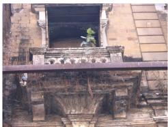
Balcony projection with bracket, balustrade in a completely neglected state
