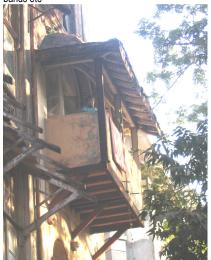
Neglected state of projecting balconies, supported on brackets with sloping roof
