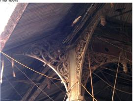
Cast iron bracket detail supporting the sloping roof
