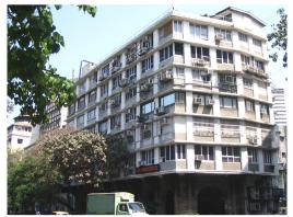
Front façade with an ground floor arcade and 3 added floors above, opening alterations etc
