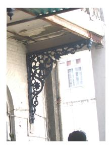
Cast iron bracket supporting the floor
