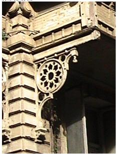
Cast iron brackets supporting the cantilevered floor
