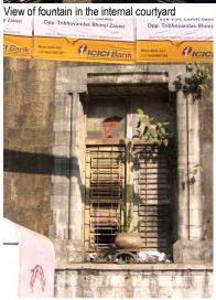
Rectangular window with band around, shutters in broken condition
