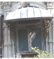
Curved awning detail on cast iron brackets
