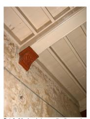
Detail of the bracket supporting the wooden roof. Wall with seepage marks due to neglected state.
