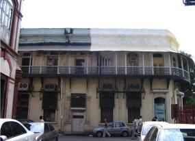
North side façade with projecting balconies supported on brackets, wooden columns and metal railing. Openings have been incongruously
