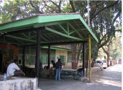
Workshop shed structure with Mangalore tiled sloping roof supported on wooden truss.
