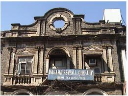
Grey stone clad building with rectangular window openings with pediments, columns with decorative capitals, round openings. The building is in a neglected state with incongruous additions.
